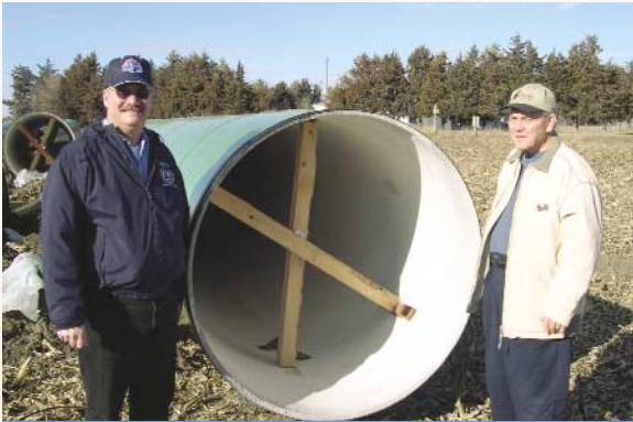
SD Assoc. of Rural Water Systems Executive Director Dennis Davis and Chairman Kuehl stand next to a section of 54" diameter pipe on RWP-2.
