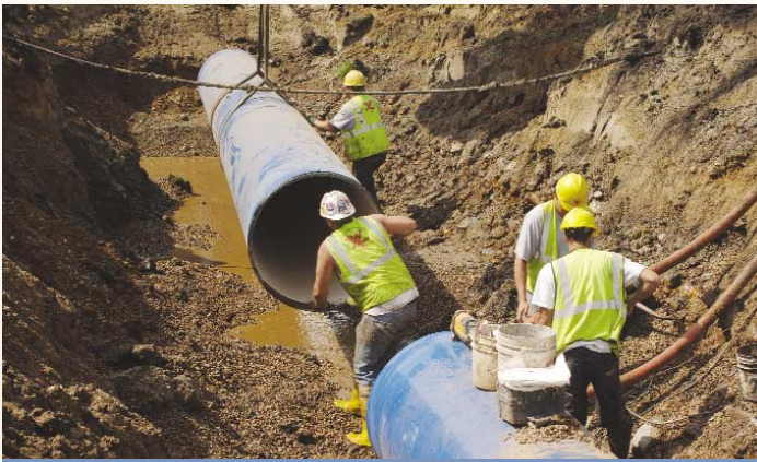
36" diameter pipe being lowered into the trench
