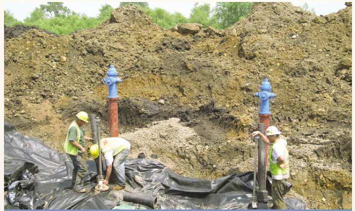
Workers install two blow off hydrants near a drainage way
