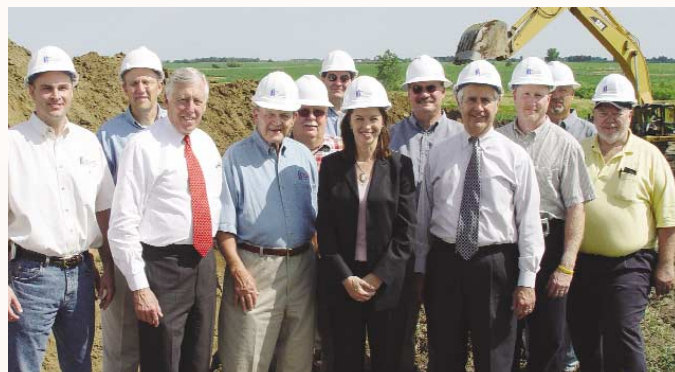
Representatives Hoyer (third from left) and Herseth (center) tour construction near Sioux Falls
