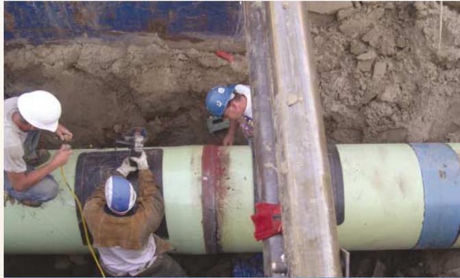
Workers in the trench weld, grind, and inspect a joint. A blue protective sleeve will be placed over the top of the joint. Note the blue sleeve to the right, which was installed as a test.
