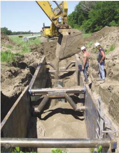
The first pipe sections being backfilled, with the next sections ready to go.
