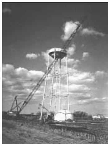
—A new water tower under construction
