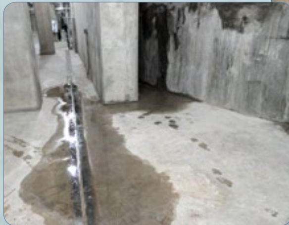
Top: Leak in one of the solids contact basins.
