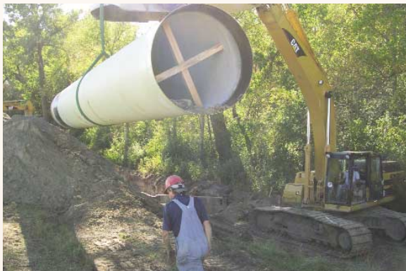
A 40 foot section of 48" diameter steel pipe being installed on RWP-1
