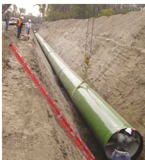
Push-on joint pipe being lined up on RWP-2
