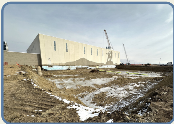
Excavation for two more solids contact basins
