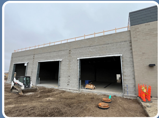
New maintenance area
