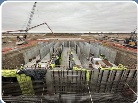
Construction of the three-million gallon underground clearwell
