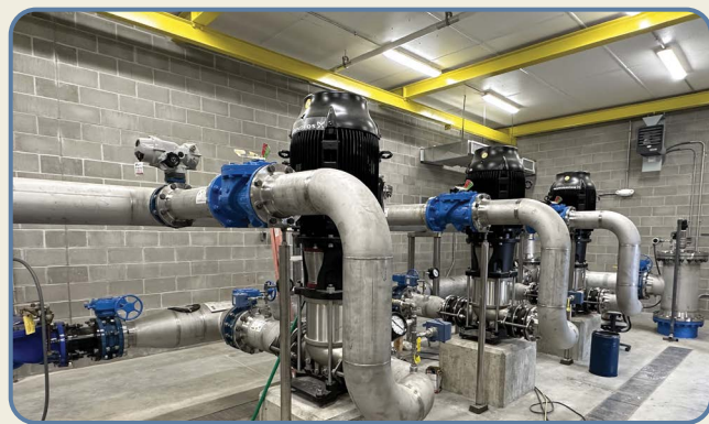
Hull pump station process piping and pumps
