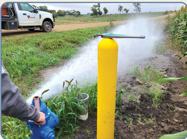
Halme flushing a portion of the line
