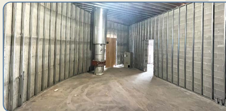
Interior masonry wall and metal studs at Beresford
