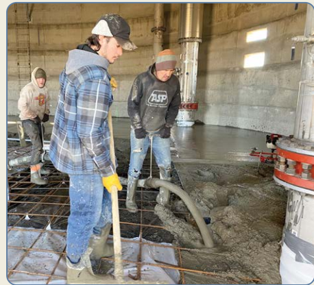
Floor being poured at Beresford
