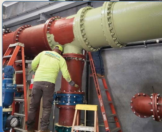
Process piping being painted
