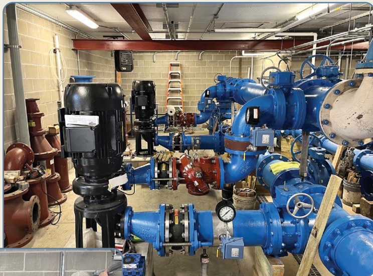
Motors and VFDs being installed at pump station
