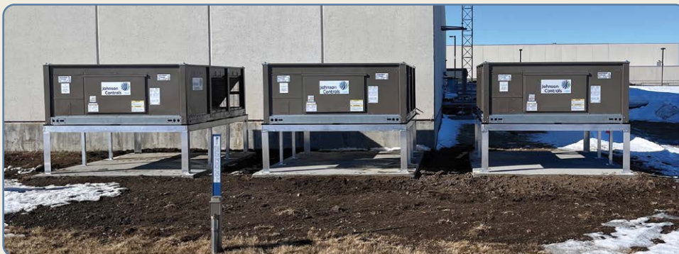
A/C units installed to replace the ineffective louvers in cooling the high service pump station
