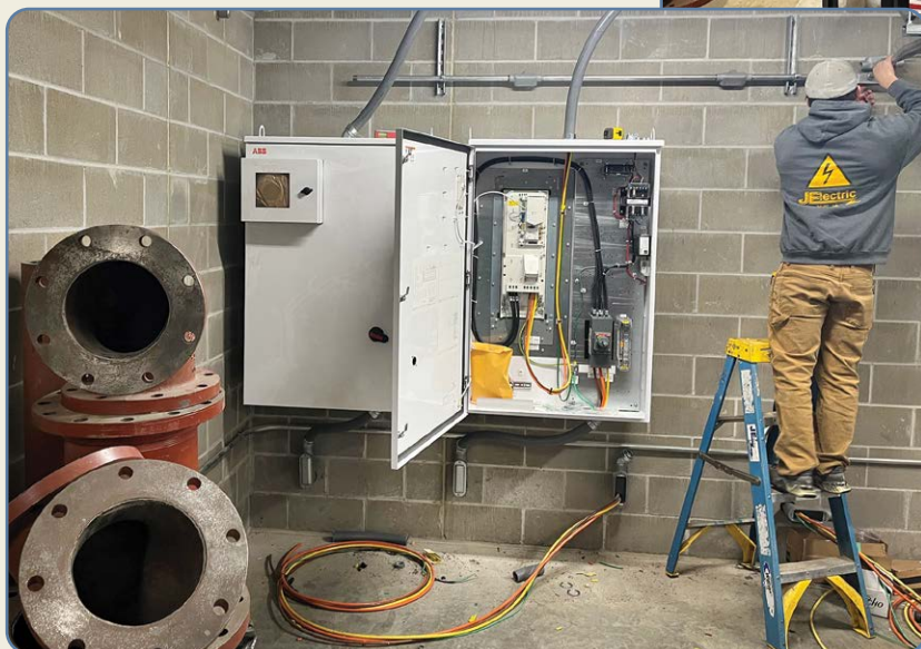
Motors and VFDs being installed at pump station
