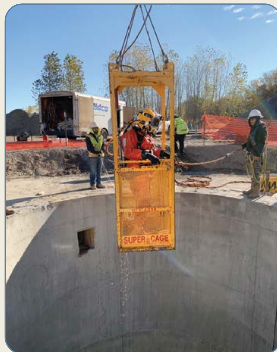
Above: Divers were used to set steel beams at the bottom of the caisson and help pour the slab of concrete for the floor
