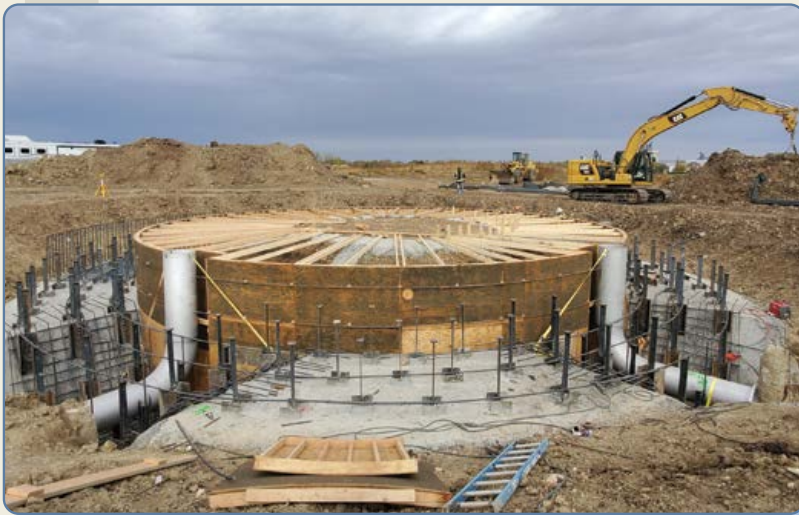
Influent pipe on the left and effluent pipe on the right
