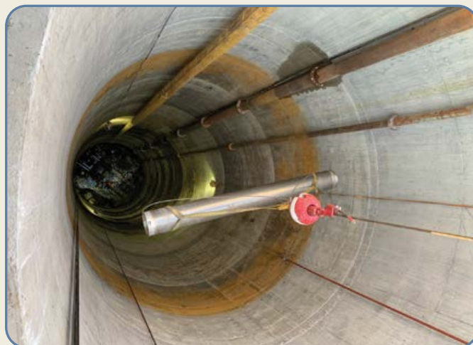
Below: 10-foot section of screen is lowered into the caisson
