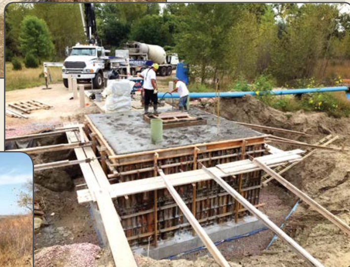
Above and Right: Work on a vertical well vault
