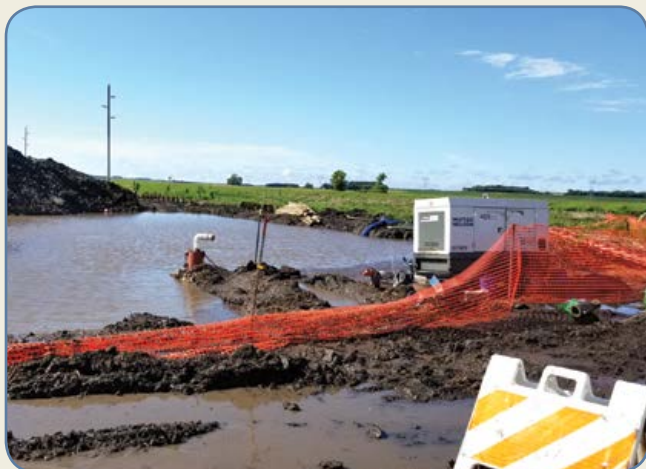
Bore pit that flooded multiple times
