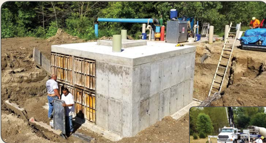
Above and Right: Work on a vertical well vault
