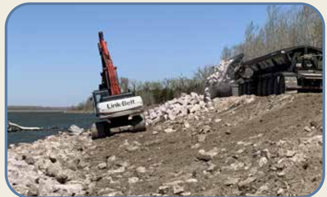
Revetment repairs in 2021
