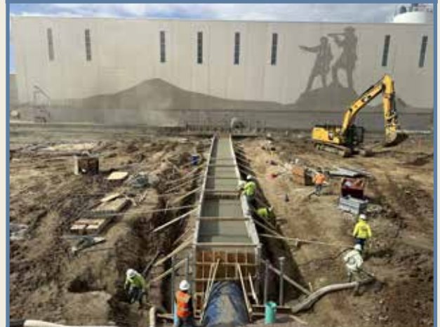
Concrete encasement of the 54-inch raw water line
