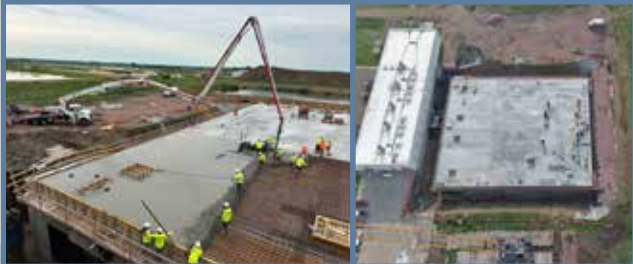
Clearwell top slab
