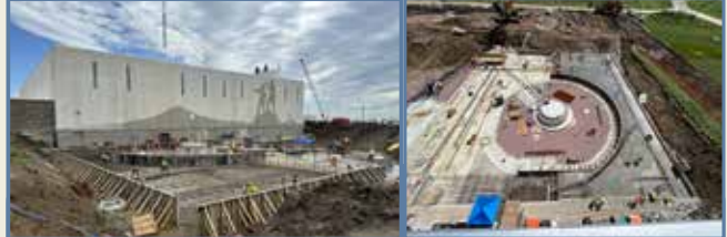
Placing rebar and pouring concrete for the base slab for the west solids contact basin
