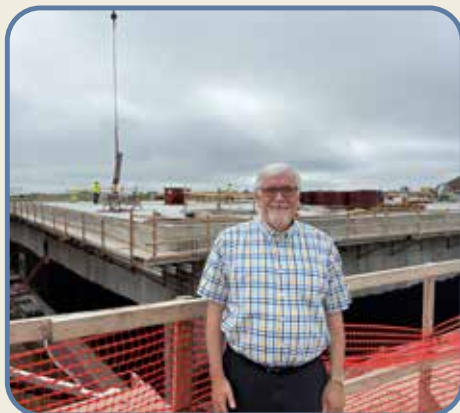
Long-time congressional aide Chuck Ackman from Senator Amy Klobuchar's office toured the water treatment plant and construction on June 27
