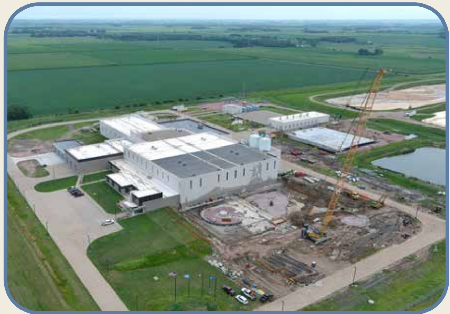
Placing rebar and pouring concrete for the base slab for the west solids contact basin
