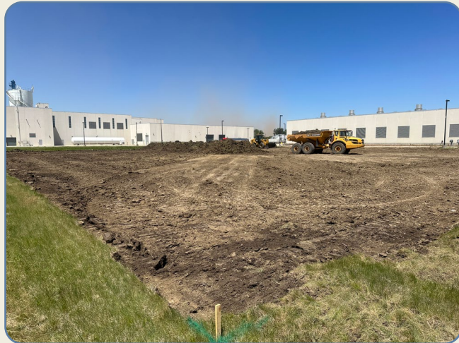
Dirt work begins for the second clearwell
