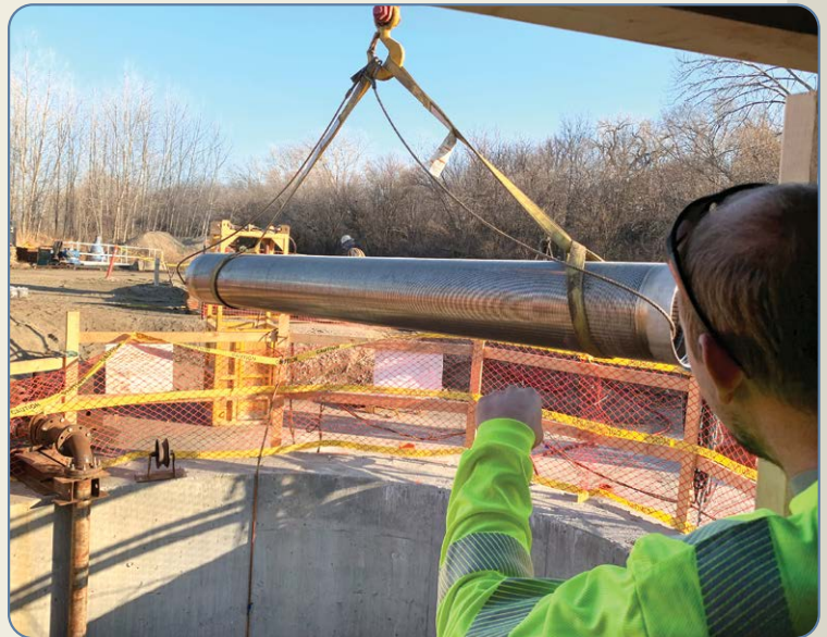
Ten-foot section of screen being lowered into the collector well caisson
