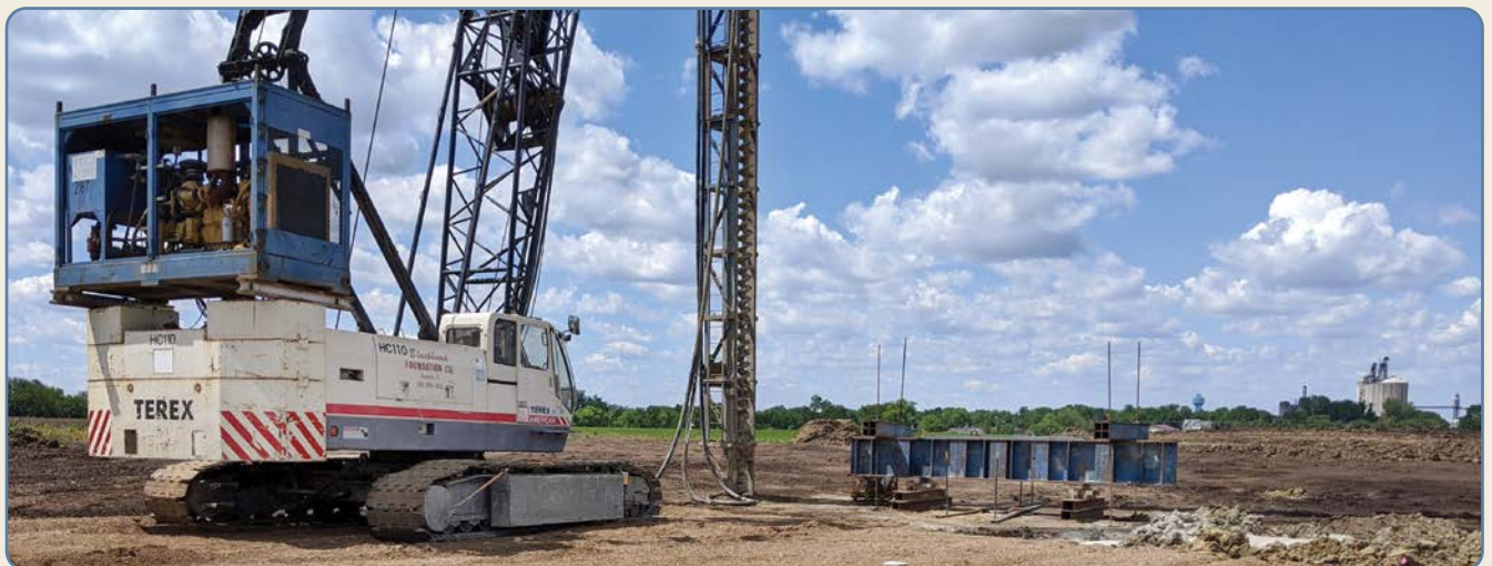
Drilling a piling outside of Beresford using the auger cast system before work was halted
