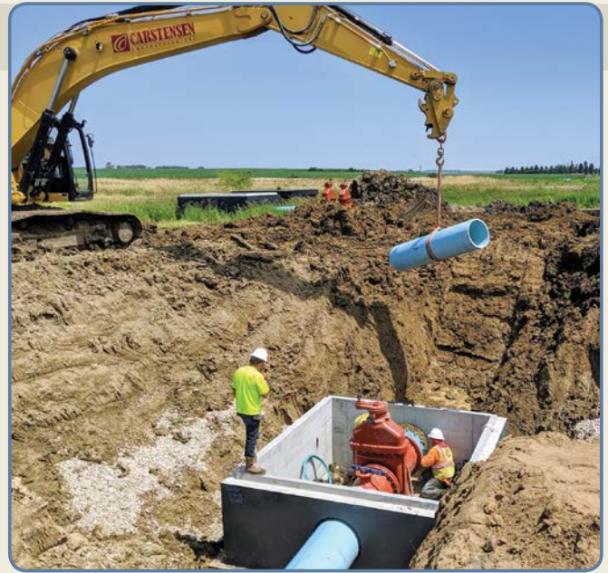
Isolation valve vault and pipeline construction
