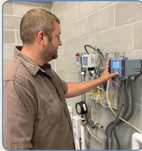
Distribution Operator Justin "JD" Walsh calibrates a pH analyzer at the MCWC-East meter building
