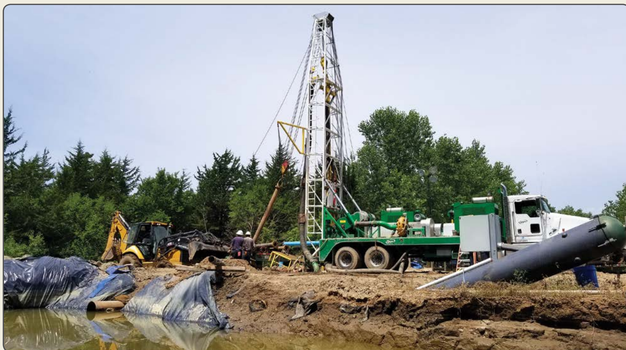
Below: Vertical well being drilled. The adjacent angle well being replaced is in the lower right hand corner.
