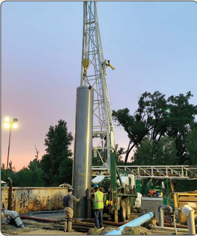
(Left and right): 36 inch screen being lowered into wells
