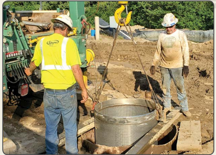
(Left and right): 36 inch screen being lowered into wells
