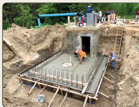
Above: Concrete being poured for a new vertical well vault, which utilizes the adjacent vault from an abandoned angle well. The circle in the center is the temporary cover for the new well.
