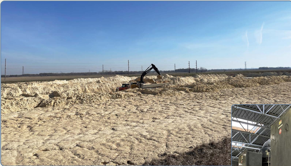
Gacke Enterprises started removing sludge from the north drying bed in April. Each of the three existing drying beds get cleaned out every three years on a rotation basis. Lime sludge is dried down for application on farm fields.
