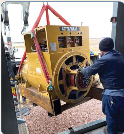
Power generator unit being removed from the backup generator
