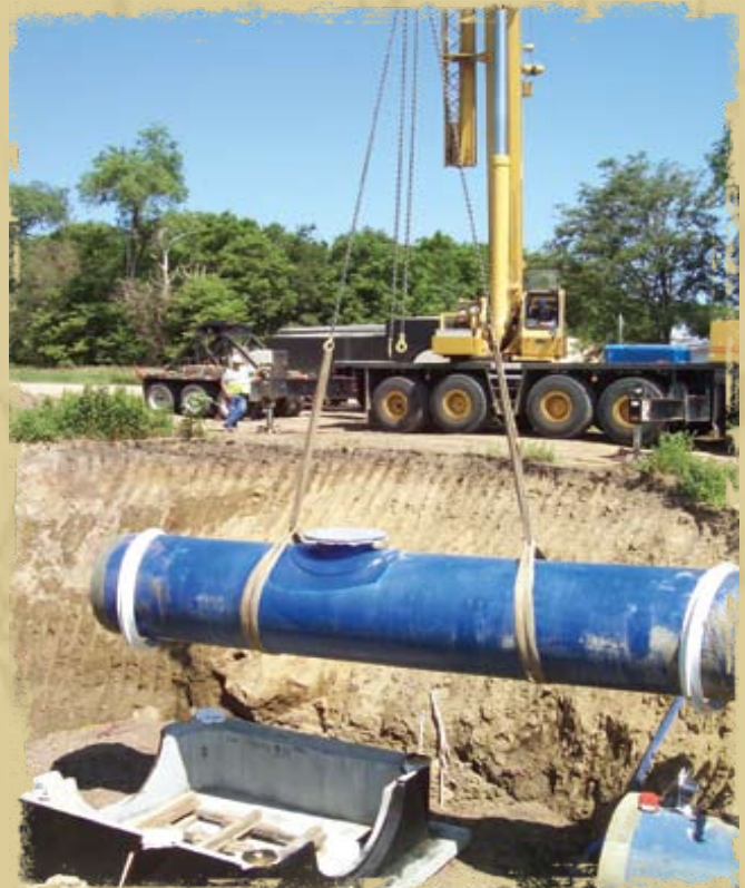
DKC lowering a 50' section of 54" pipe onto an air release valve vault with a 100 ton crane near the Vermillion River.
