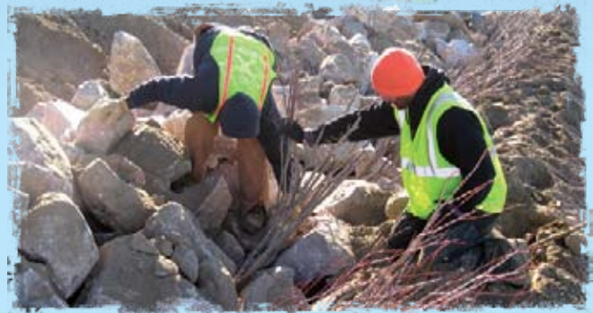
Workers planting willow trees in December 2007 before the revetment was covered with soil. The photo below shows a current view of the bank stabilization.
