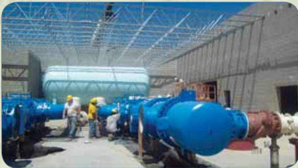
Roof going up over surge tank (background) and pipe gallery.
