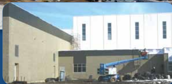
Metal paneling being installed on administrative area.
