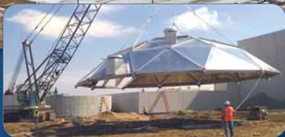
Aluminum dome being installed on the gravity thickener.
