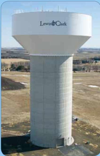
The water tower holds three million gallons and stands 190' tall.
