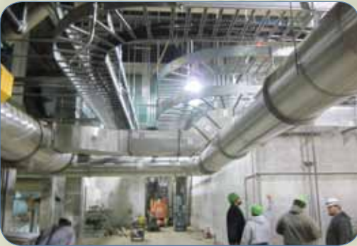
Electrical cable trays and duct work.
