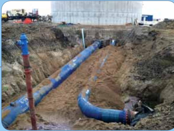
24" piping connecting the transmission line with the piping in the base of the water tower.
