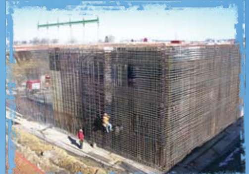
Mats of rebar being placed for the 3' thick walls of the wetwell.
