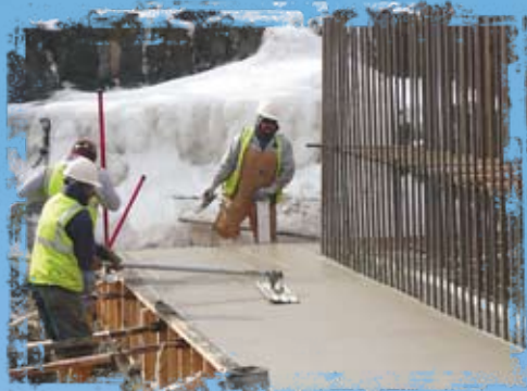
2' thick concrete floor for the wetwell.
