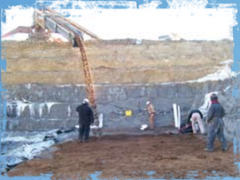
Covering the under drain system of the wetwell with select fill materials.
