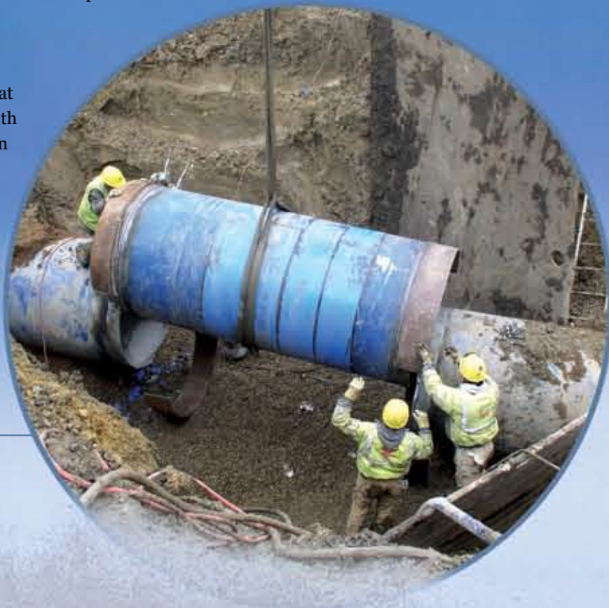
Last section of pipe being installed on TWP-5, connecting it with a previously completed segment of the main transmission line.
