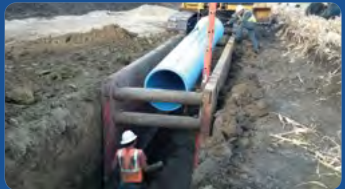
Using a trench box for pipe construction
