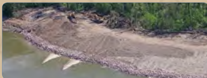
Repair of the "stone toe"
