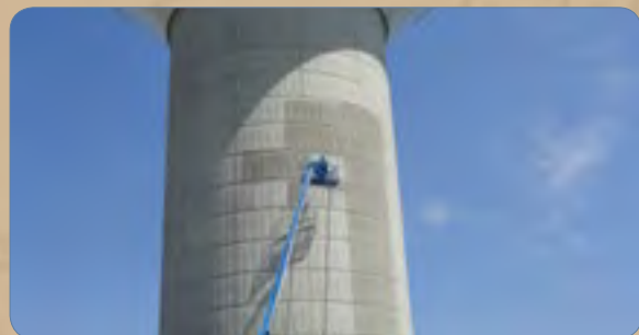
Sandblasting the concrete pedestal
