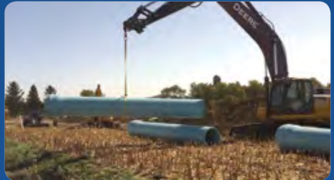
First section of 30" PVC pipe being installed
