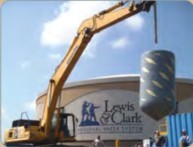
One of two "pigs" used during disinfection of main trunk line.
