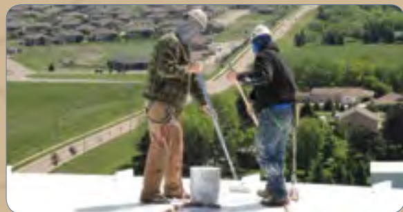
Painting the top of the water tower
