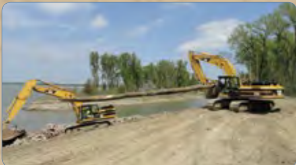
Locked log being moved into place
