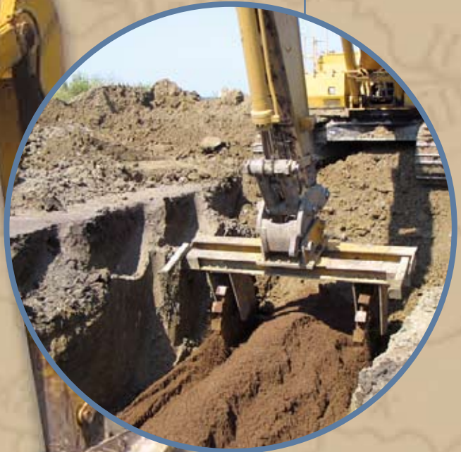
Segment 5: Trench packing
