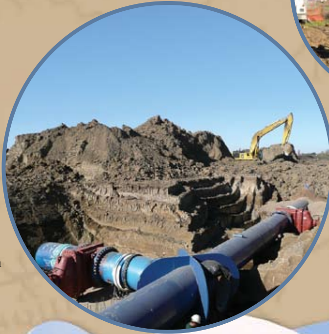
Segment 6/7A: Turnouts and valves for future pump station near Beresford.
