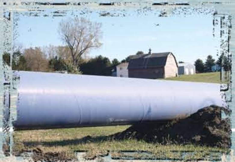
Pipe laid out near Lennox on Segment 5.
