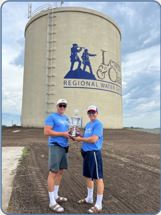
DN Tanks reached substantial completion on the one-million gallon ground storage reservoir a few miles east of Madison on August 2 and water began flowing to Madison that day! Senate Majority Leader Casey Crabtree (left) and Greater Madison Area Chamber of Commerce Executive Director Eric Hortness taped a funny "Cool Dads" video on August 29 with Executive Director Troy Larson. It can be seen on the videos link of the Chamber's Facebook page.
