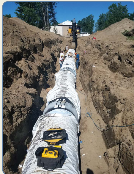
800 feet of 42-inch ductile iron pipe connects the pump house to the raw water transmission line
