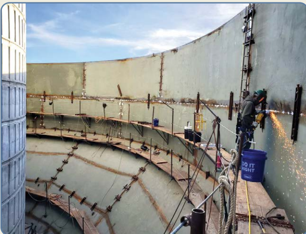
Grinding down tack welds inside the tank
