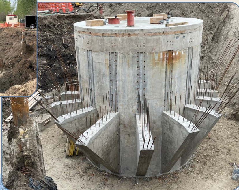
Below: Lower half of the buttresses
