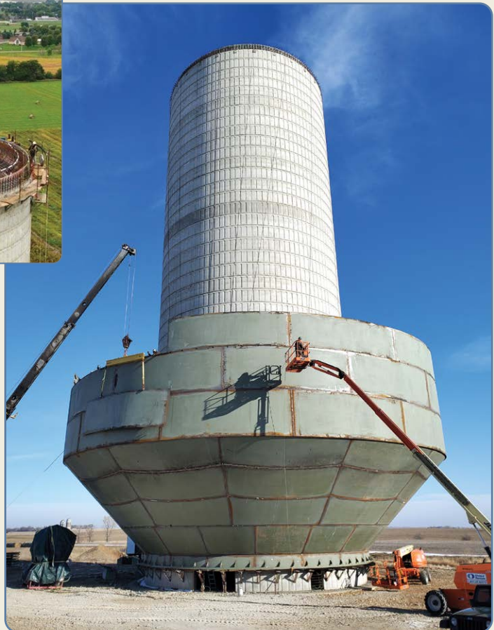
Welding the steel panels for the tank
