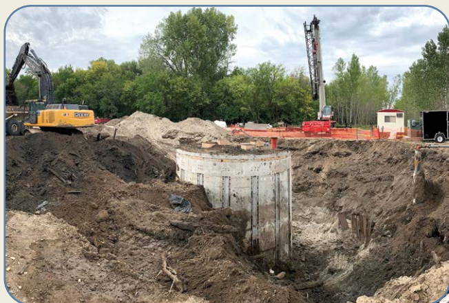
Above: Excavating for the buttresses (lots of buried stumps and trees encountered)
