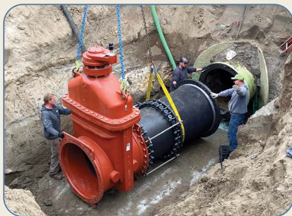
Top two photos: Tying into the raw water pipeline
