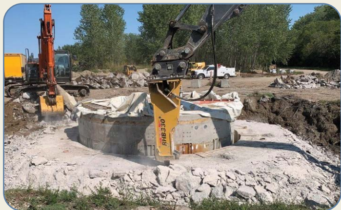
Right photo: Breaking up the "deadman" that was used to sink the caisson
