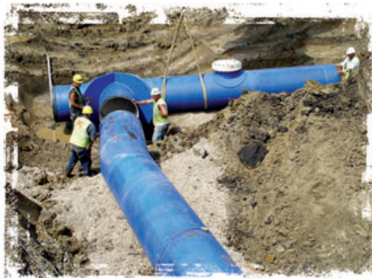
St. Louis Construction works on a joint on TWP-1 west of Sioux Falls.
