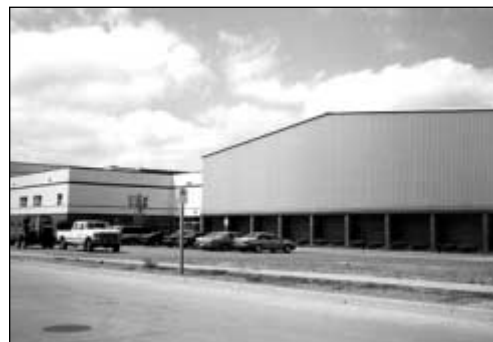
—New classroom addition at Western Christian
