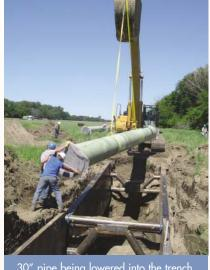
30" pipe being lowered into the trench. A "trench box" is being pulled, which narrows the area needed to be excavated.
