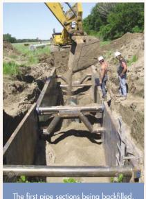
The first pipe sections being backfilled, with the next sections ready to go.
