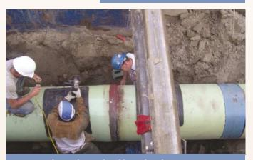
Workers in the trench weld, grind, and inspect a joint. A blue protective sleeve will be placed over the top of the joint. Note the blue sleeve to the right, which was installed as a test.
