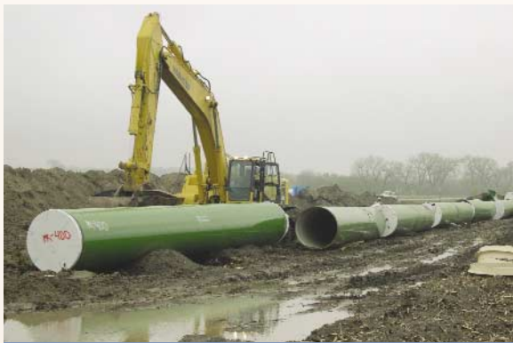
High Country Pipeline working in wet conditions near Vermillion
