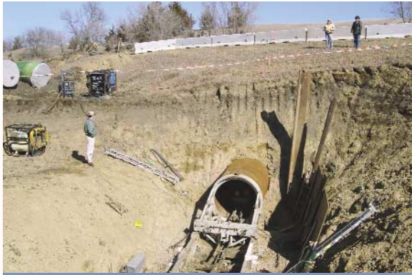
Boring of Bluff Road north of Vermillion
