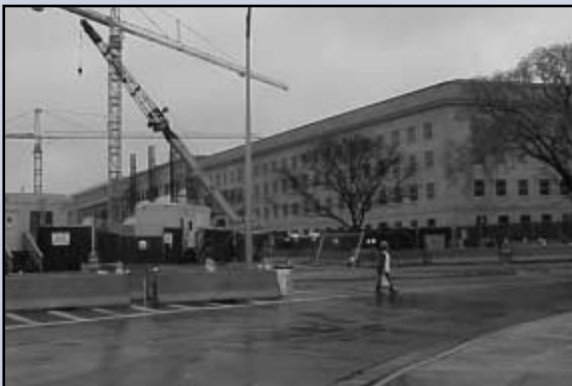
Rebuilding of the Pentagon.
