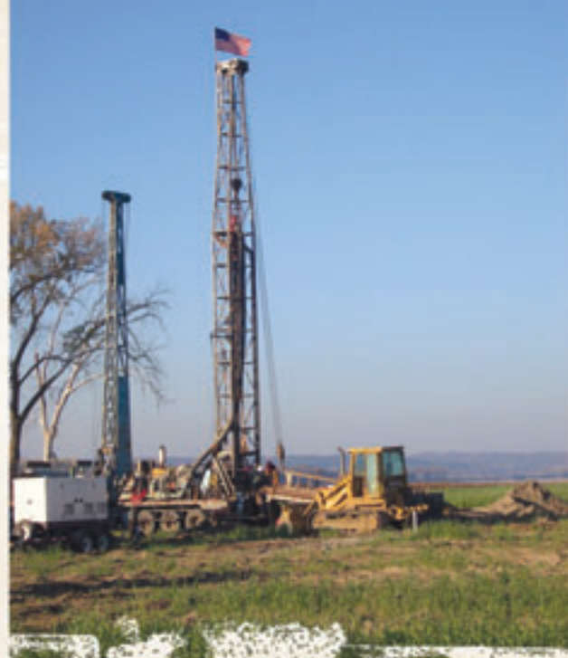
Test well being drilled at Site J
