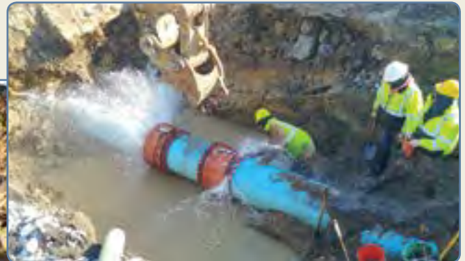
Above and Left: Repairing leaks on the 24-inch pipe
