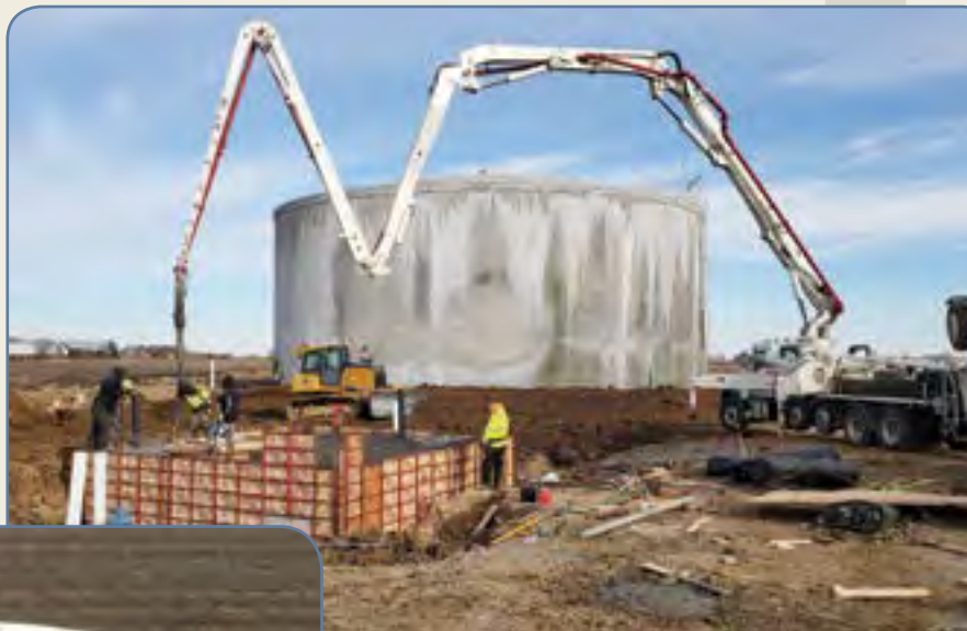
Above: Constructing the vault
