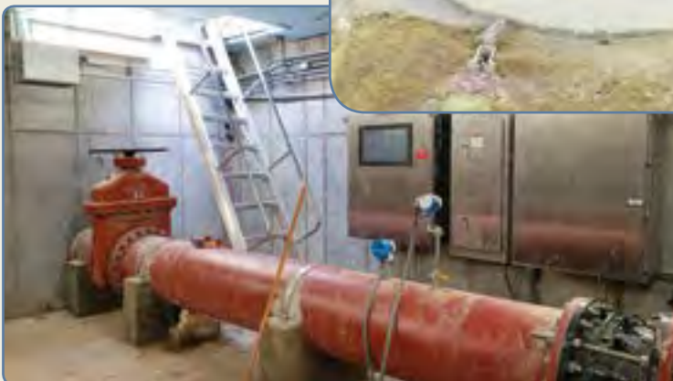
Below: Inside the vault
