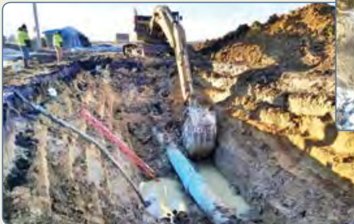
Above and Left: Repairing leaks on the 24-inch pipe
