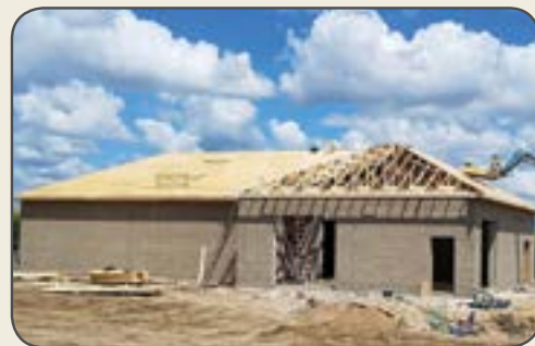
Rock County Pump Station
