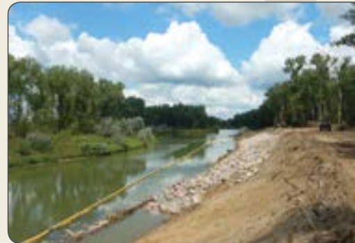
Above Right: Revetment repair Right: Revetment extension
