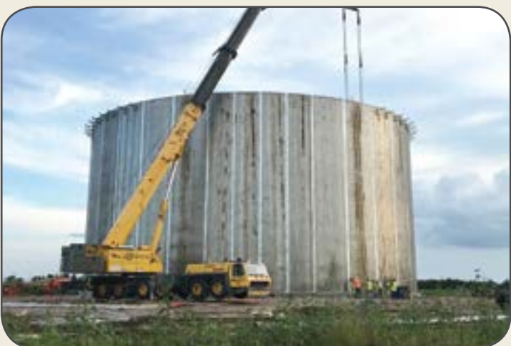
58 feet tall wall panels for the Rock County reservoir
