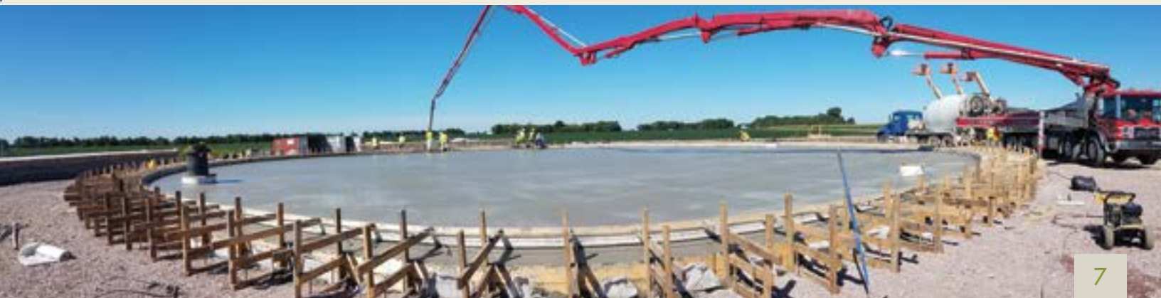
Pouring the floor for the Rock County reservoir
