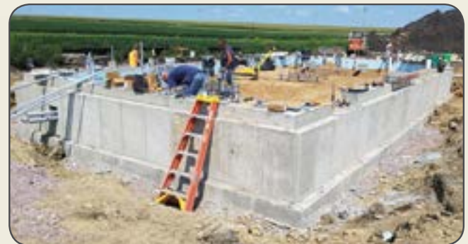
Foundation walls for the Adrian meter building
