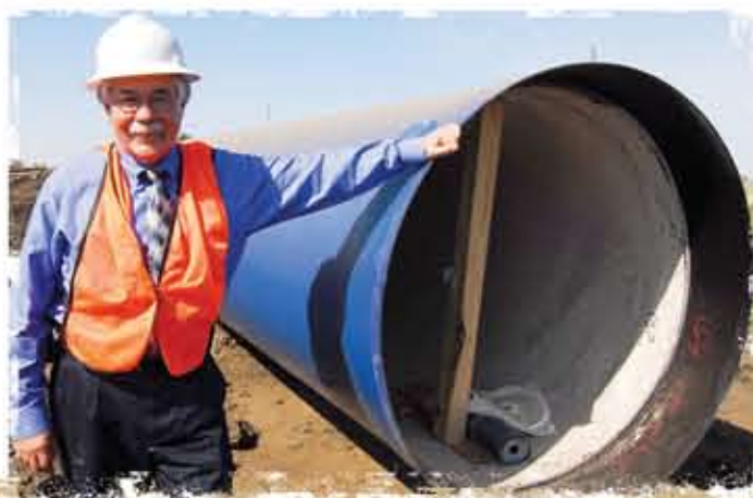
Reclamation Commissioner Johnson sizes up a section of 54" pipe.
