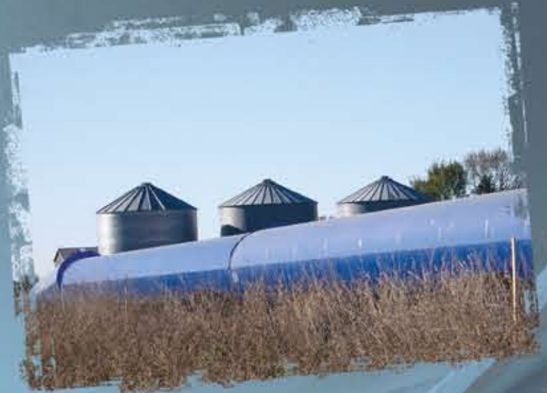
54" pipe laid out along TWP-5.
