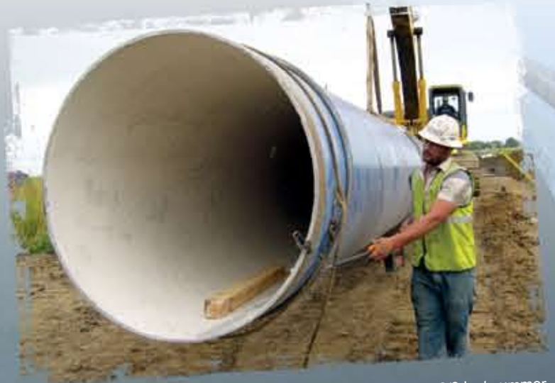
"Holiday testing" the coating on a 54" section of pipe on TWP-2/3 last summer.
