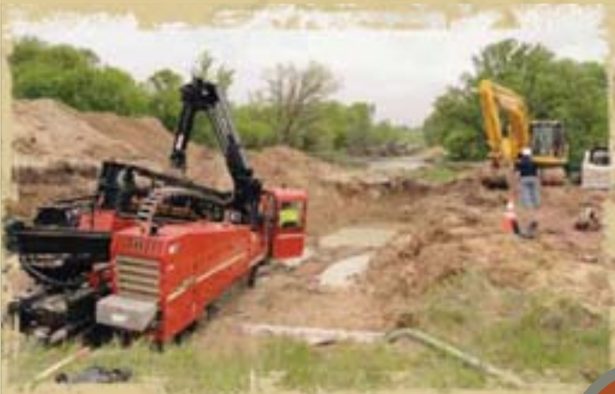
Directionally drilling under the Big Sioux River.
