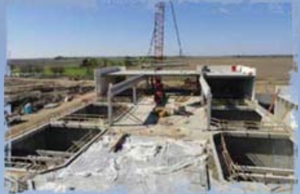
Roof beams going up over the filter area.
