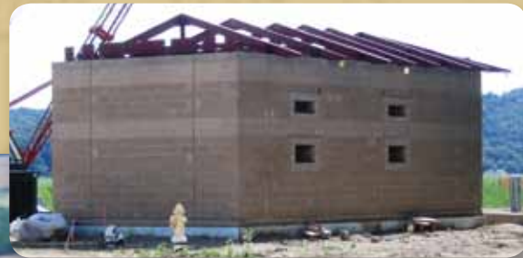
Roof going up on well/pump house at Well Site E.
