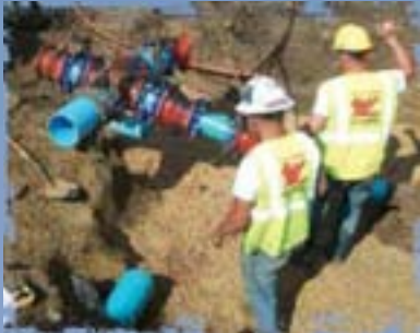
Making the connection with Beresford's infrastructure on TWP-11.
