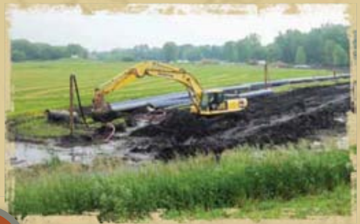
Contractor "de-watering" on the SD side of the Big Sioux River.
