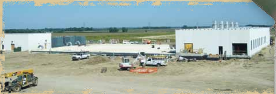
Below: Electrical switchgear building & three standby generators (left), three million gallon underground reservoir (middle) & pump station (right).
