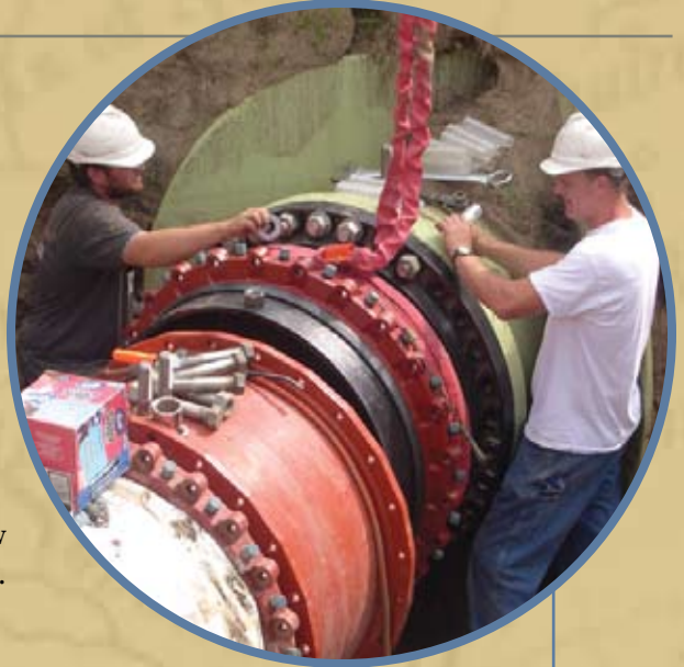
The last section of well piping being connected to the raw water pipeline.
