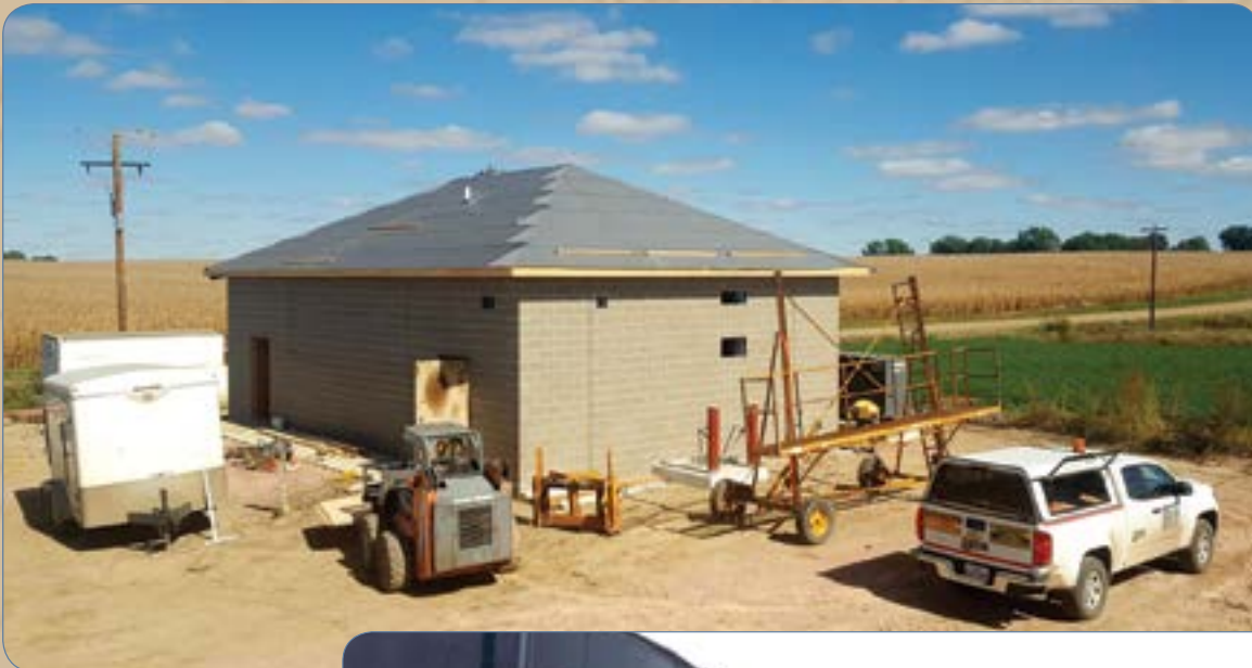
Crooks meter building/ pump station
