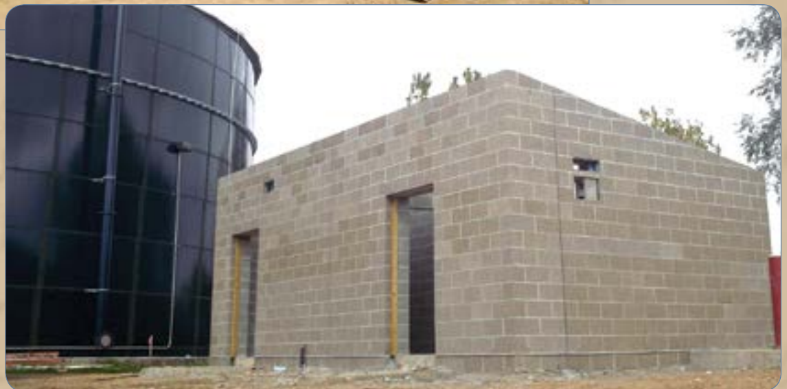
Madison meter building
