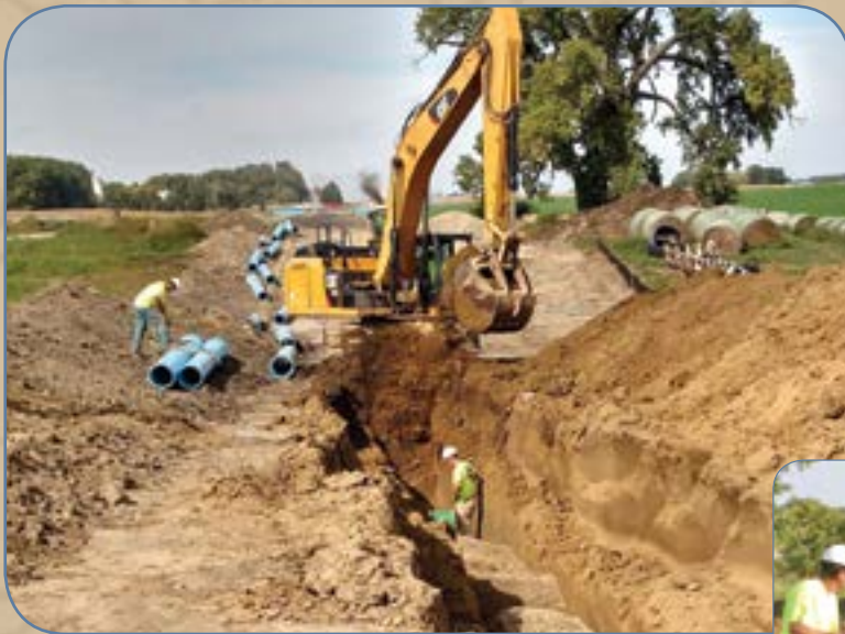
Installation of 16-inch pipe
