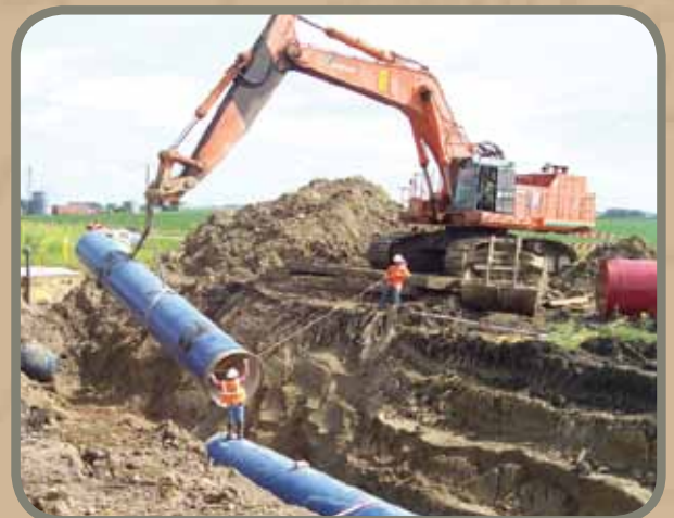
The last 50' long section of 54" pipe being lowered into the trench.
