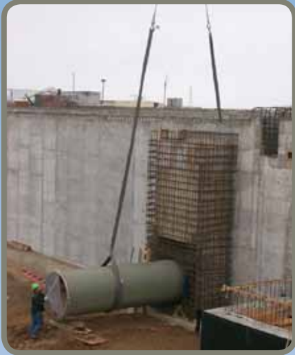
54" diameter pipe being installed into the clearwell.
