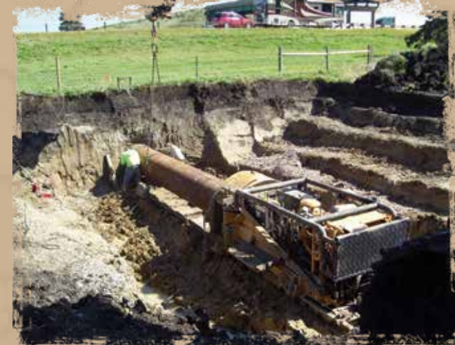
Boring under I-29 west of Beresford.
