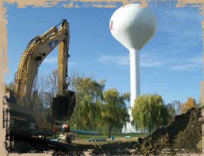
8" PVC pipe being installed for the Lennox service line.
