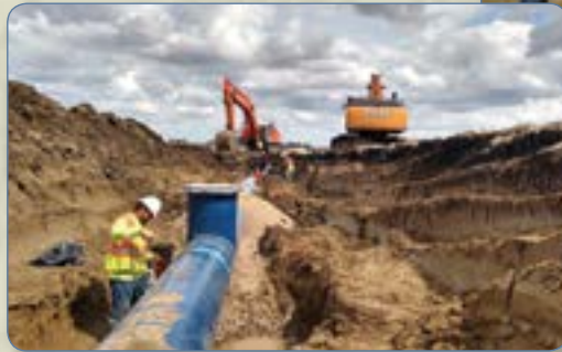
Manway provides access to inside of pipe during construction
