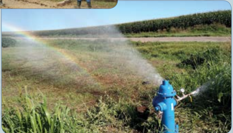
Below: Pressure testing the 14 inch Luerne service line
