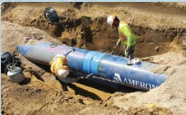
Canusa wrap is put on joints to add further corrosion protection
