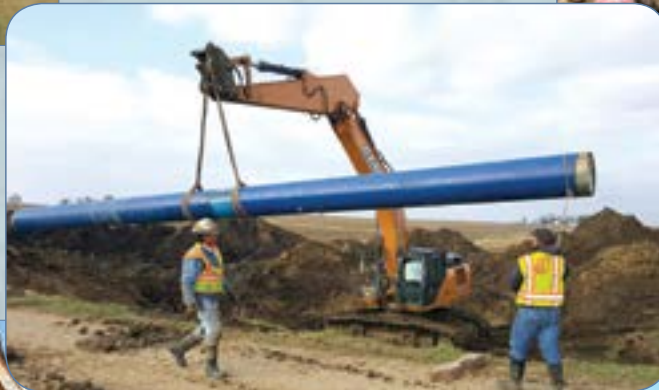
Left: Last section of 24 inch pipe being installed
