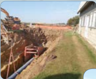
Above: Working in a narrow easement area
