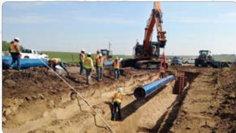
First section of 24” steel pipe
