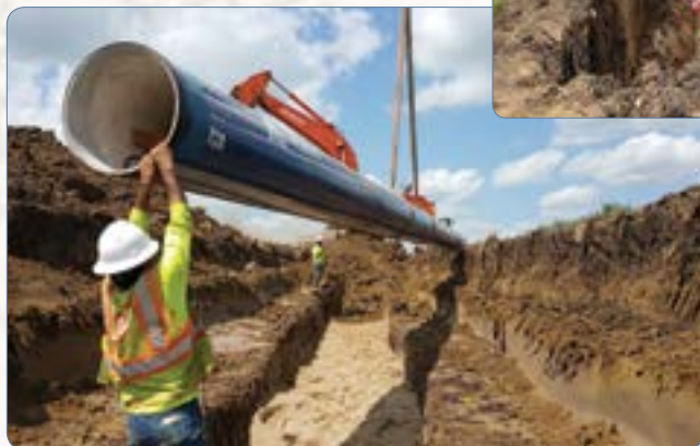
Section of 24” pipe being lowered into the trench
