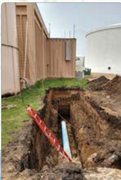
First section of 24” steel pipe
